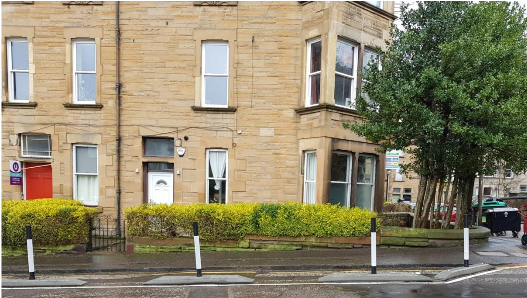
View of 112 Viewforth ( white door ) Boundary wall to be rebuilt. Trees and hedge to be removed
